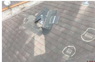
Wind damaged shingles at two story residence in McAllen, TX.
